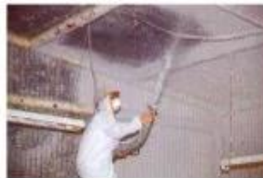
Structural steel and deck coating
