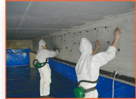
INJECTION "Asbestrip"
